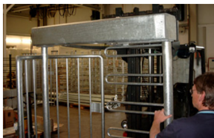
Fig. 9: Mounting the support beam
