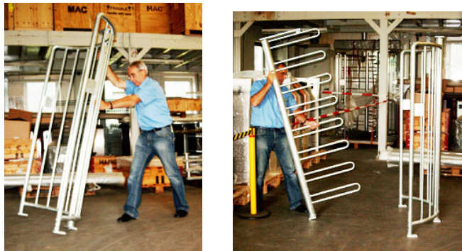
Fig. 7: Setting up Cage halves and guide combs
